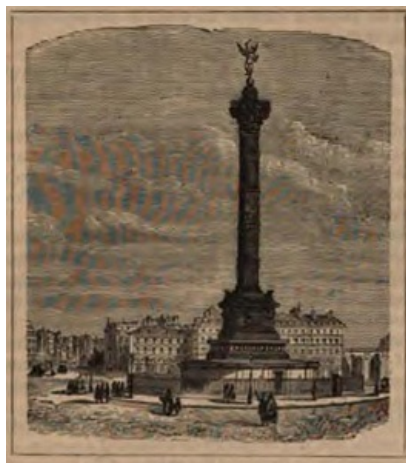
Column of July, Place de La Bastille.
