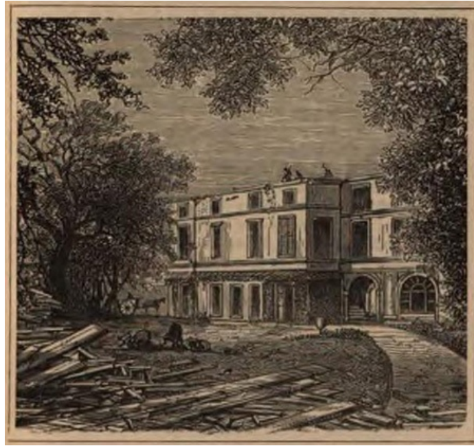
House of M. Thiers During Demolition and Removal.
