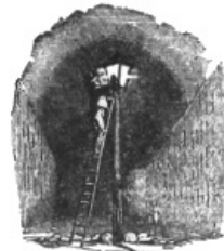
A Man lighting a Gas-lamp.
