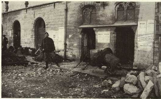
When the Germans had finished with Termonde, the bells in the tower of the burned Hôtel de Ville crashed to the pavement
