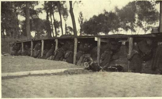
The defence of Termonde. Belgian infantry firing from trenches built with head-covers as a protection from shrapnel
