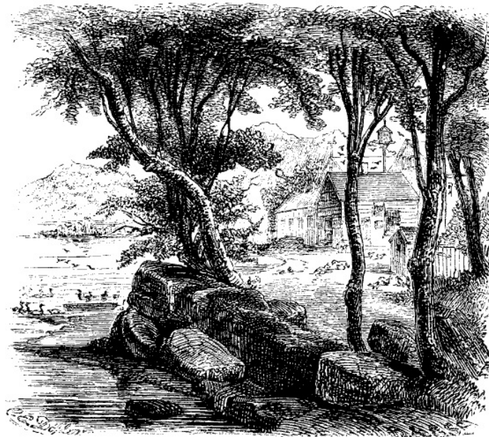
THE MILLMAN'S HOUSE.
