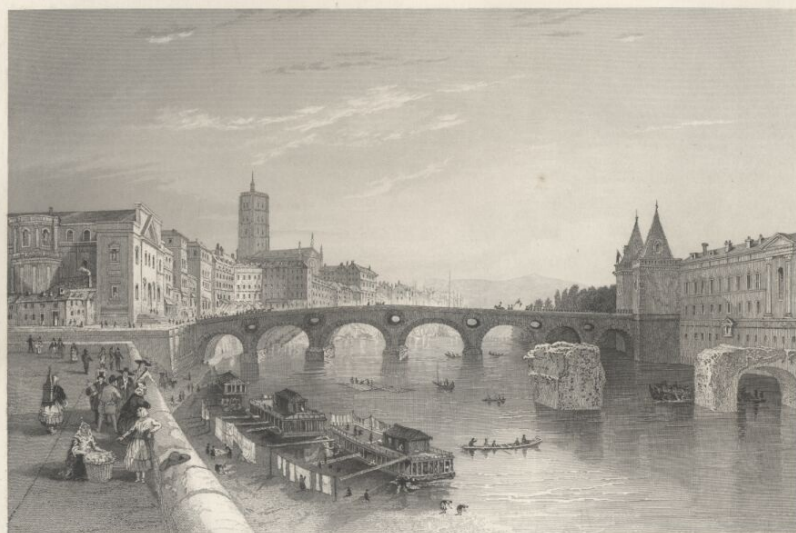
THE BRIDGE OF TOULOUSE.
