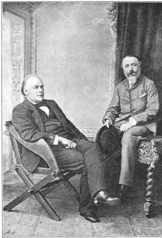
From a photograph by T. Westley, 57, Vernon Street, Northampton. CHARLES BRADLAUGH AND HENRY LABOUCHERE.
