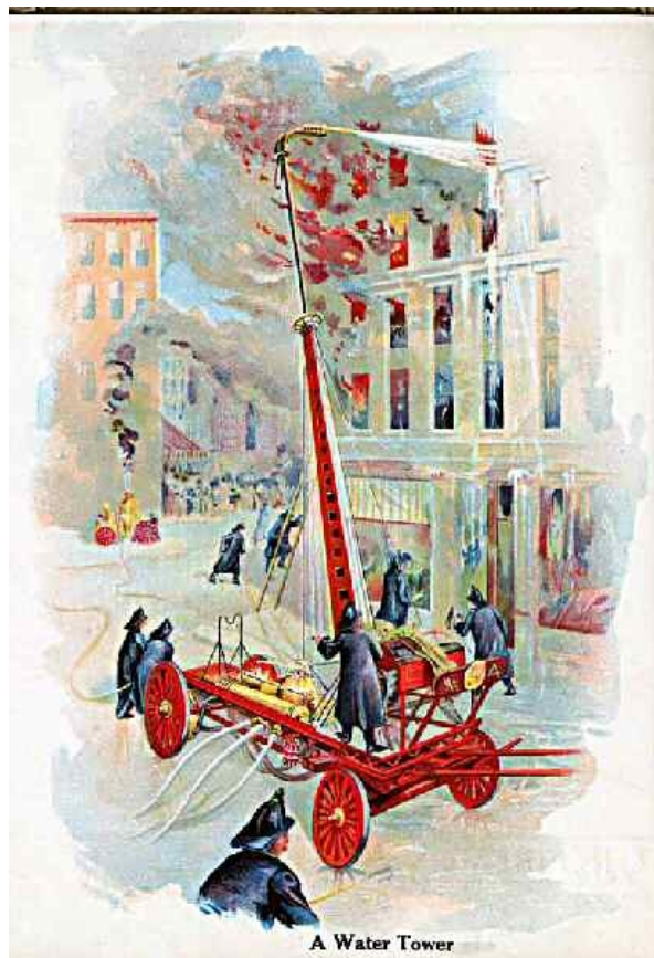
A Water Tower
