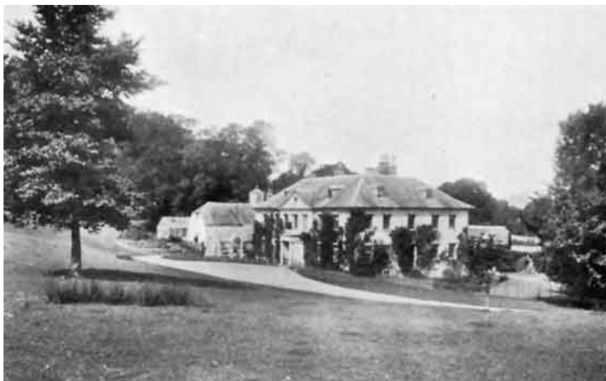
Alfoxden House, Near Holford
