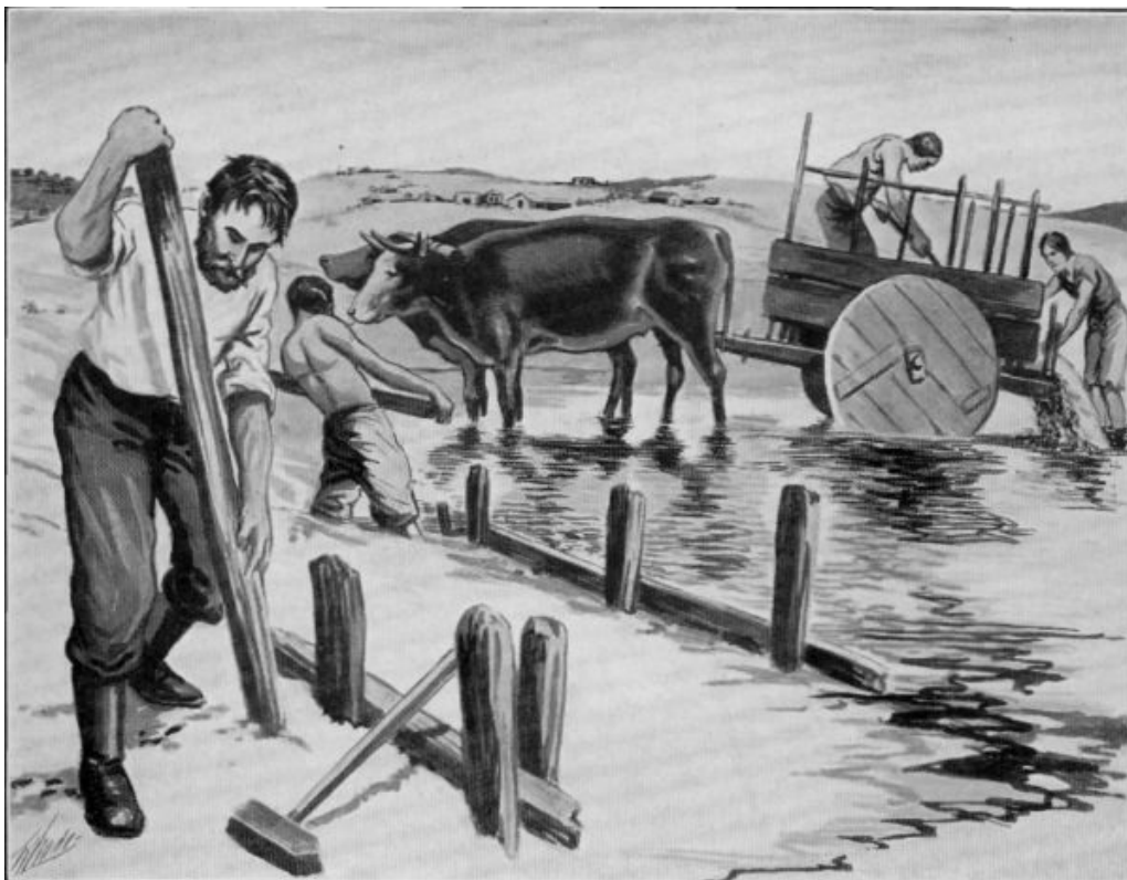
Men with shovels, leveling the sand-hills, piled the wagons high with shimmering grains which were ... dumped into pile-surrounded bogs. San Francisco reached farther and farther out into the bay.
