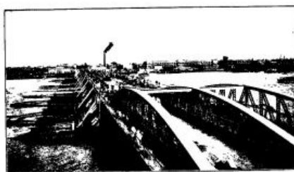
Photo. 191 Howrah Bridge from Calcutta side. Publication of Aliphetra
