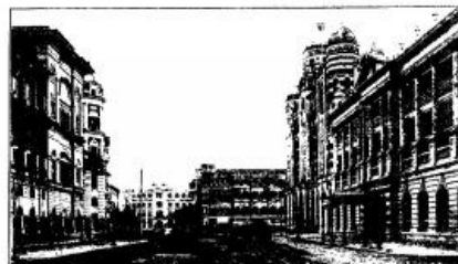
Present view of Clive Street, showing Chartered Bank's premises on the right, middle centre. [P. 4. 4.]
