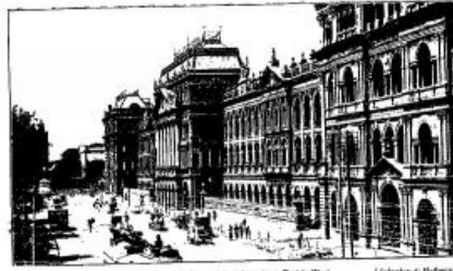
Frontage of Writers' Buildings from East to West.
