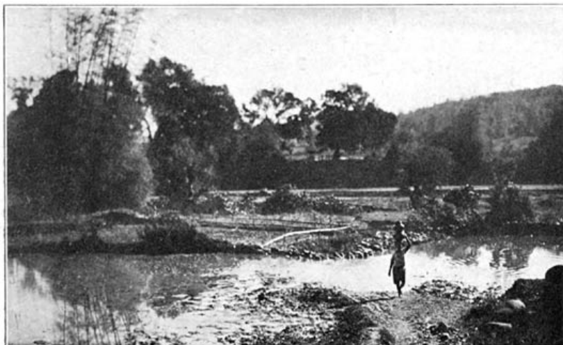
Bringing water from the stream
