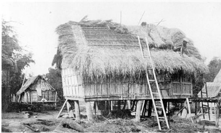
Roofing a House.
