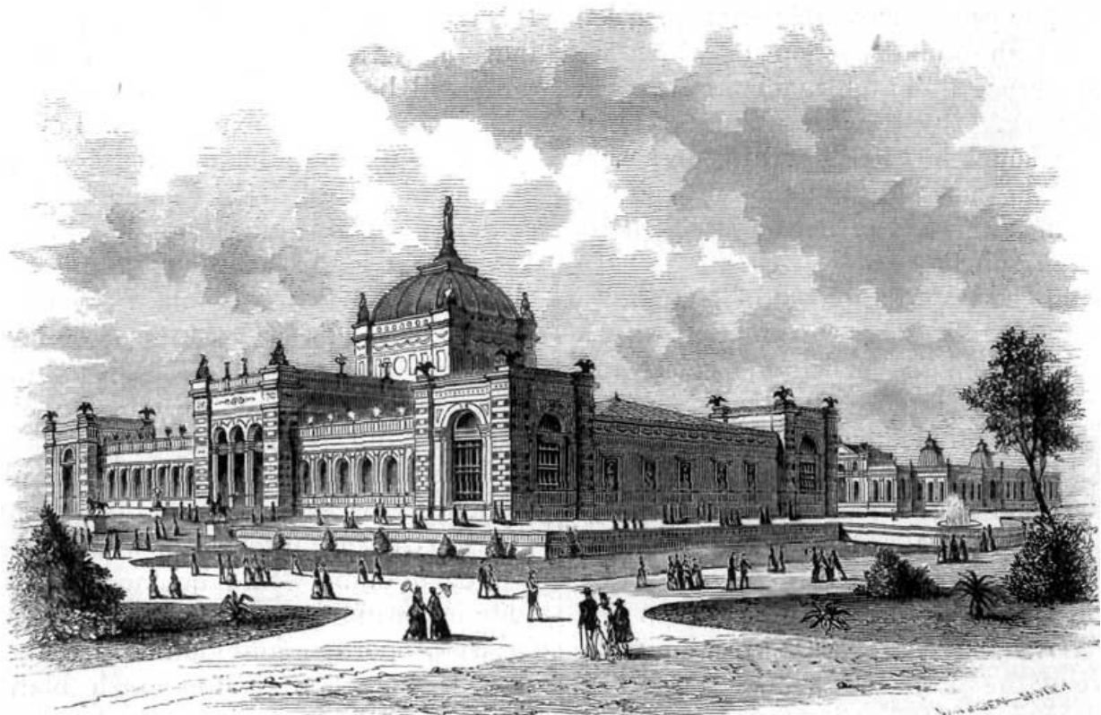
MEMORIAL HALL, WITH EXTENSION.
