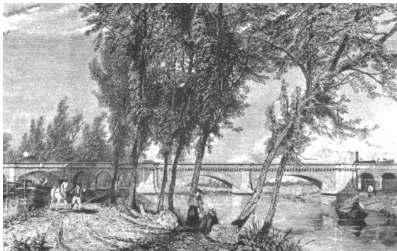
THE WARRINGTON VIADUCT, over the River Mersey and Irwell Canal.
