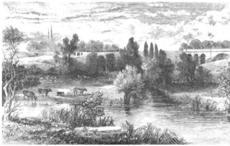
THE SHERBORNE VIADUCT NEAR COVENTRY, and Bridge over the Holyhead Road.
