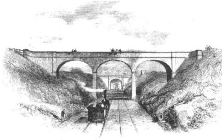
EXCAVATION AT HARTFORD.
