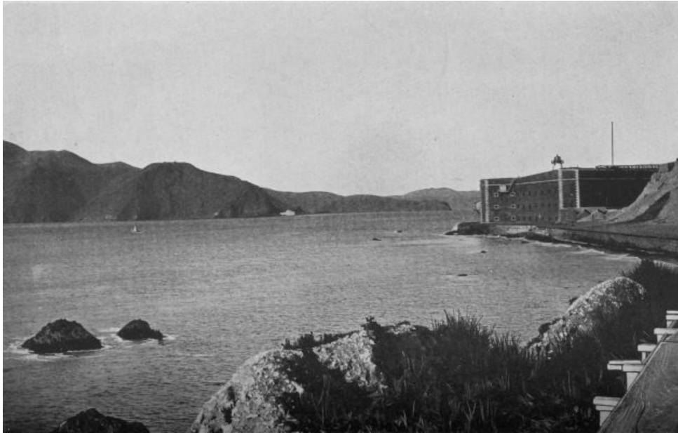
Fort Point at the Golden Gate
