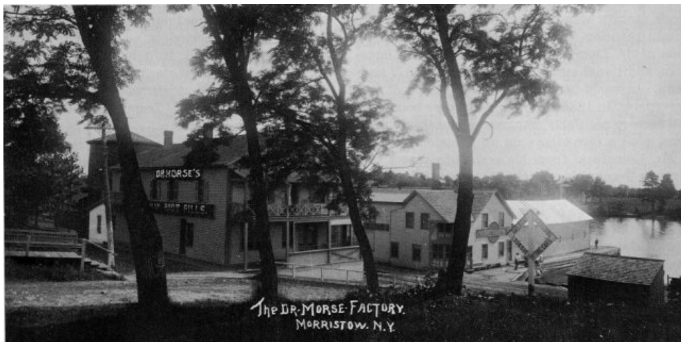
FIGURE 13.—Comstock factory buildings, about 1900.
