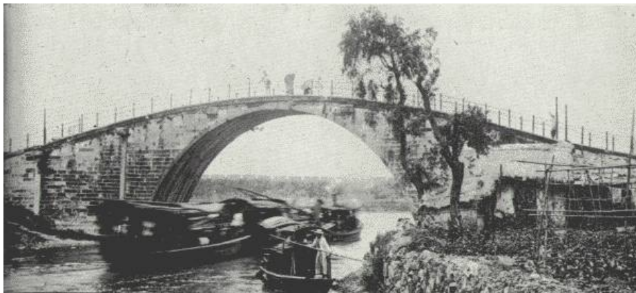
TYPICAL SINGLE-SPAN BRIDGE OF INLAND CHINA. Engineers say that China possesses bridges of more varied design than any other country.
