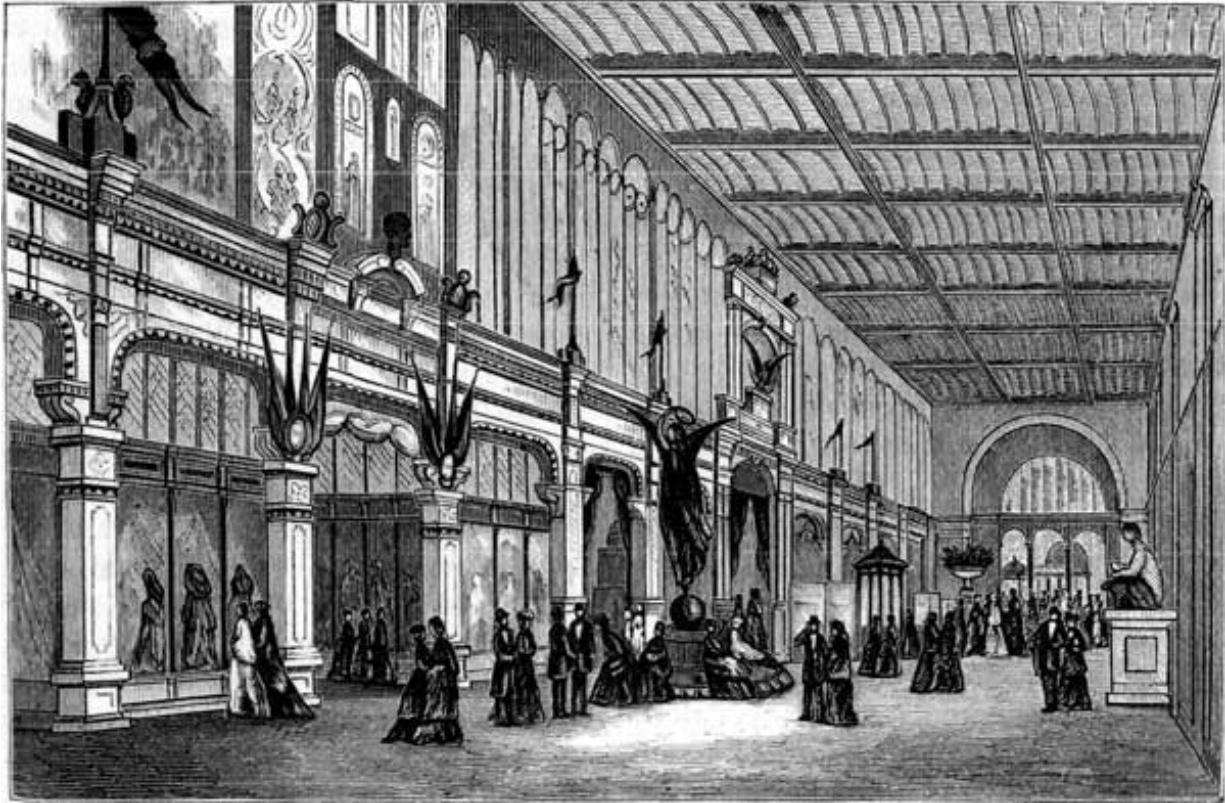
GRAND VESTIBULE OF THE PARIS EXPOSITION BUILDING, 1867.
