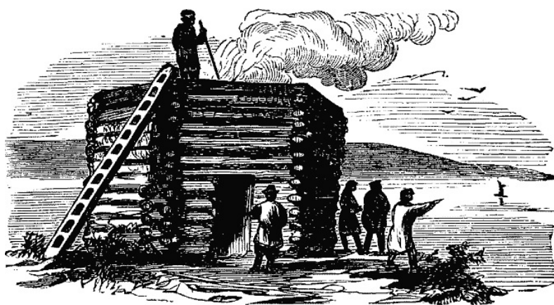
LIGHT-HOUSE AT GHIJIGA.
