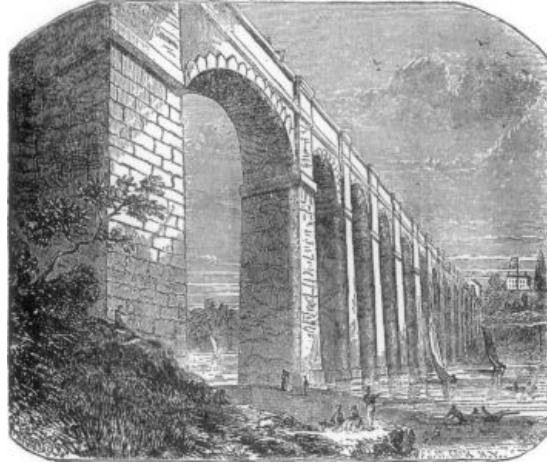
High Bridge, Croton Aqueduct
