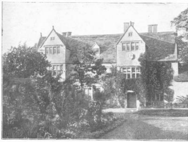
ARMSCOT MANOR HOUSE, WORCESTERSHIRE
