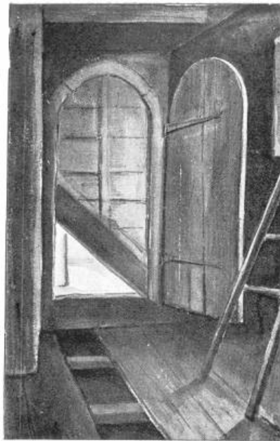
HIDING-PLACE, TRENT HOUSE
