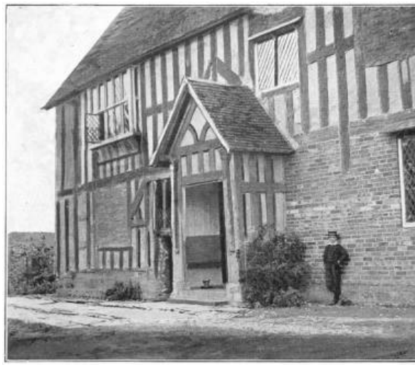
ENTRANCE PORCH, HUDDINGTON COURT
