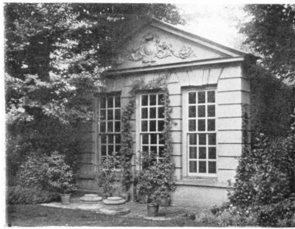
OLD SUMMER HOUSE, SALISBURY (SHOWING CARVING IN WHICH IS A PEEP-HOLE FOR HIDING-PLACE BEHIND)
