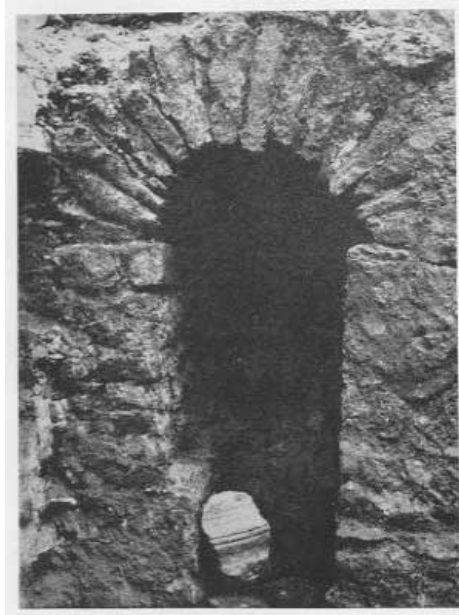
FIG. 28. LINCOLN. SEWER UNDER BAILGATE
