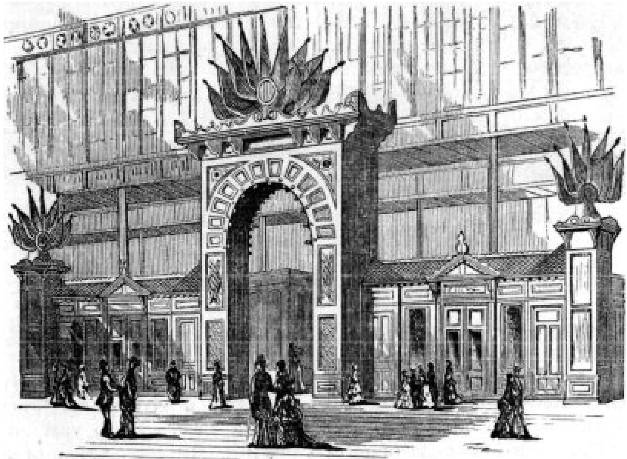
FAÇADE OF THE SWEDISH DIVISION, MAIN BUILDING.
