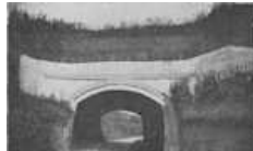
BRIDGE CARRYING THE CANAL OVERHEAD.
