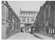
ABBEY GATE, ABINGDON, SHOWING ALL THAT NOW REMAINS OF THE ABBEY.
