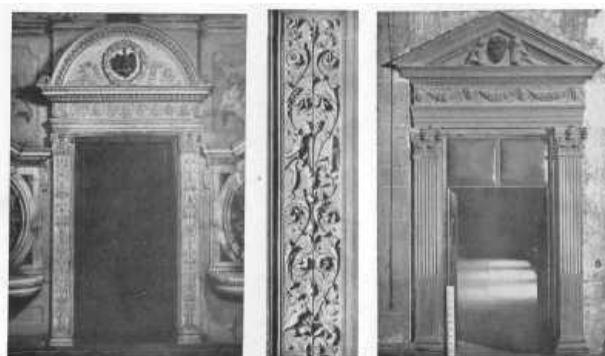
The Italian Renaissance is still inspiring the world. In the two doorways the use of pilasters and frieze, and the pedimented and round over-door motifs are typical of the period.
