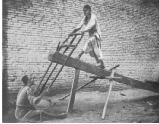
SAWING A BEAM.
