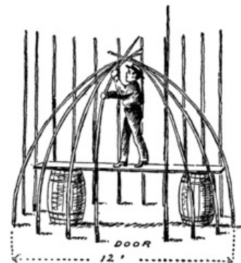
Fig. 131. Making the Frame of the Straw Hut.
