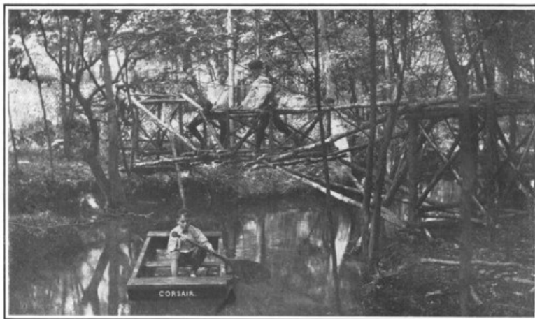
Building the Cantilever Bridge over Cedar Brook.
