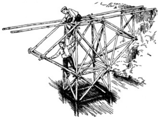
Fig. 319. Preparing to Put an E Frame in Place.
