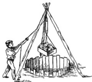
Fig. 282. Digging the Well.
