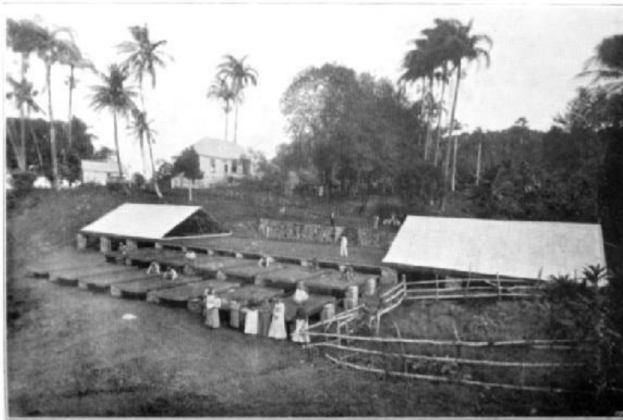
Grenada, B.W.I.: Samaritan Estate (Showing trays which slide on rails; the iron covers slide over the whole in case of wet.)
