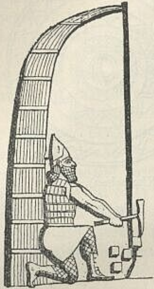
Soldier undermining a wall, sheltered by gerrhon .
