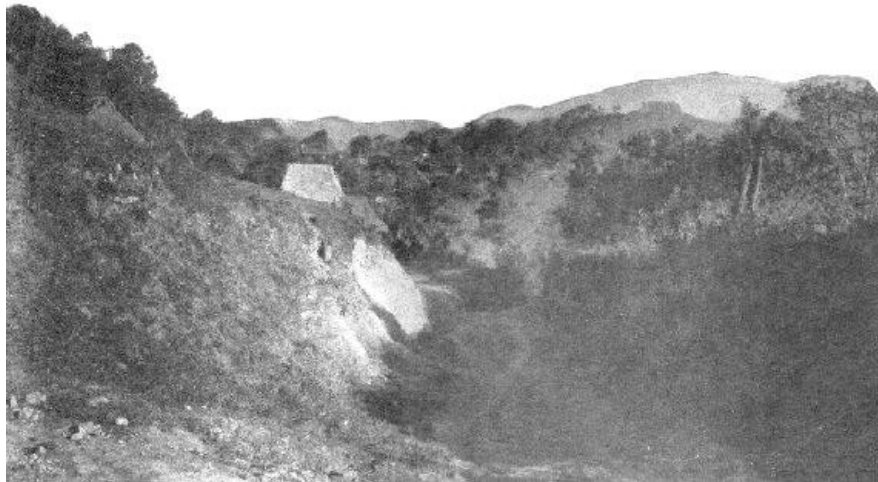
ROAD APPROACHING QUEZALTEPEC
