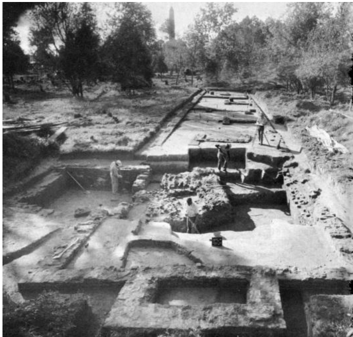
EXCAVATED FOUNDATION OF A LATE 17TH-CENTURY PROTOTYPE OF THE BALTIMORE AND PHILADELPHIA ROW HOUSES. SIX FAMILIES COULD HAVE LIVED HERE.
