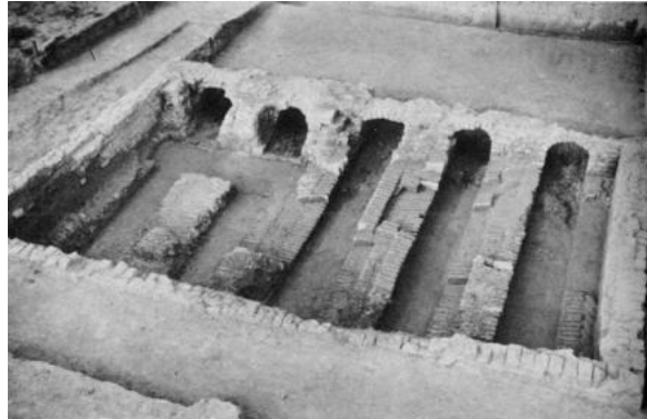
FOUR BRICK KILNS HAVE BEEN EXCAVATED. THE ONE SHOWN HAD FIVE FIRING CHAMBERS. ROOFING TILES WERE ALSO MADE IN THE JAMESTOWN BRICK KILNS.
