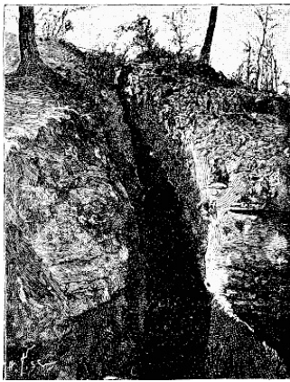
FIG. 4.—FAULT THAT CAUSED THE ACCIDENT.
