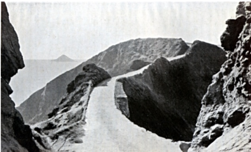
THE COUPÉE. Leading from SARK to LITTLE SARK. At the time of the story, the path was much narrower than now, there were no supporting walls, and it was continually breaking away. The pinnacles of the buttresses were also much higher. The Island to the left is LE TAS or L'ETAC.
