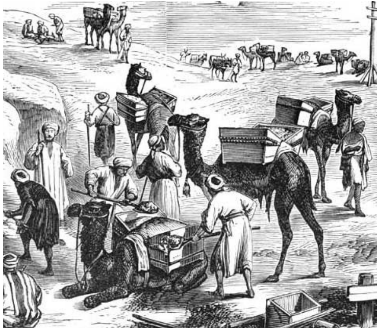
REMOVING THE EARTH FROM THE CANAL BY MEANS OF DROMEDARIES.
