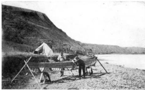
THE "ATOM I" UNDER CONSTRUCTION.
