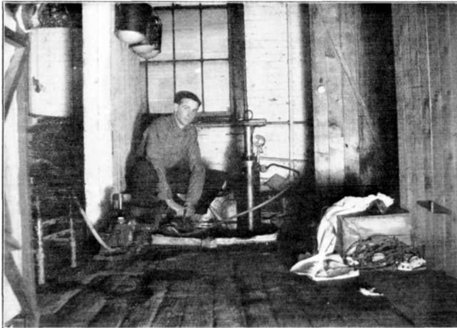
PLATE XXVIII, FIG. 1.—APPARATUS FOR MEASURING LOSS OF PRESSURE IN SUBAQUEOUS MATERIALS.
