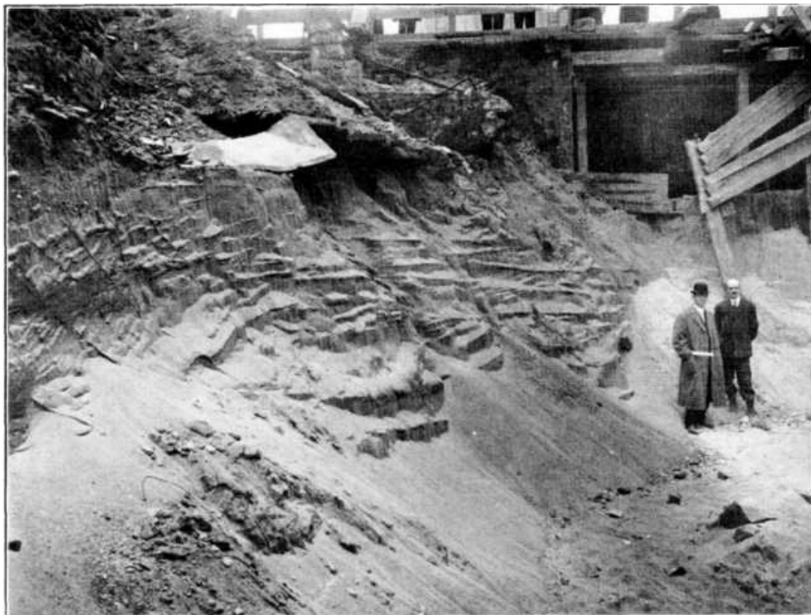
PLATE XXV, FIG. 1.—NORMAL SLOPES AND STRATA OF NEWLY EXCAVATED BANKS.
