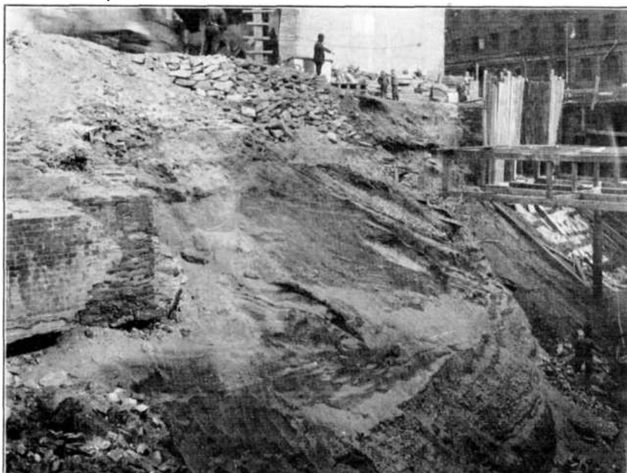
PLATE XXV, FIG. 2.—NORMAL SLOPES AND STRATA OF NEWLY EXCAVATED BANKS.
