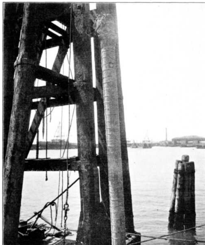
PLATE XXIX, FIG. 2.—CHENOWETH PILE, PENETRATING HARD MATERIAL.
