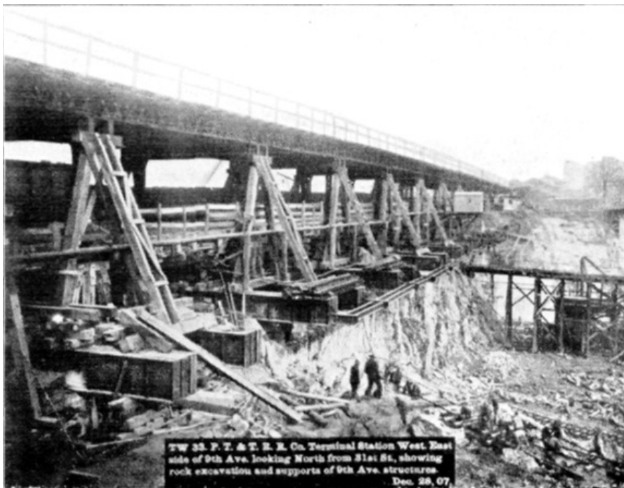
PLATE XLVIII, FIG. 1.— TW 33, P.T. & T.R.R. CO. TERMINAL STATION WEST. EAST SIDE OF 9TH AVE. LOOKING NORTH FROM 31ST ST., SHOWING ROCK EXCAVATION AND SUPPORTS OF 9TH AVE. STRUCTURES. DEC. 28, 07.
