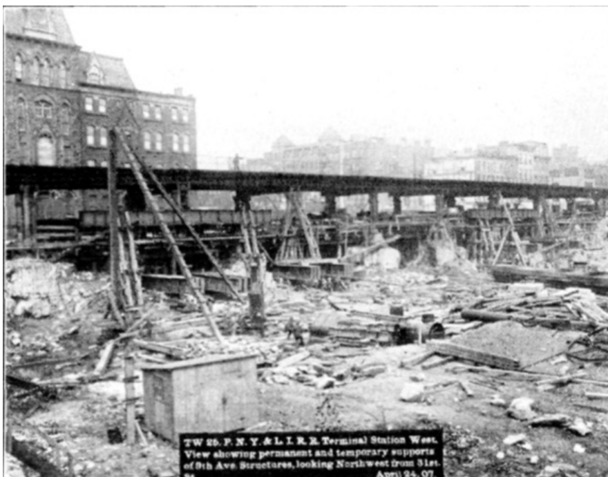
PLATE XLVII, FIG. 3.— TW 25, P.N.Y. & L.I.R.R. TERMINAL STATION WEST. VIEW SHOWING PERMANENT AND TEMPORARY SUPPORTS OF 9TH AVE. STRUCTURES, LOOKING NORTHWEST FROM 31ST. ST. APRIL 24, 07.
