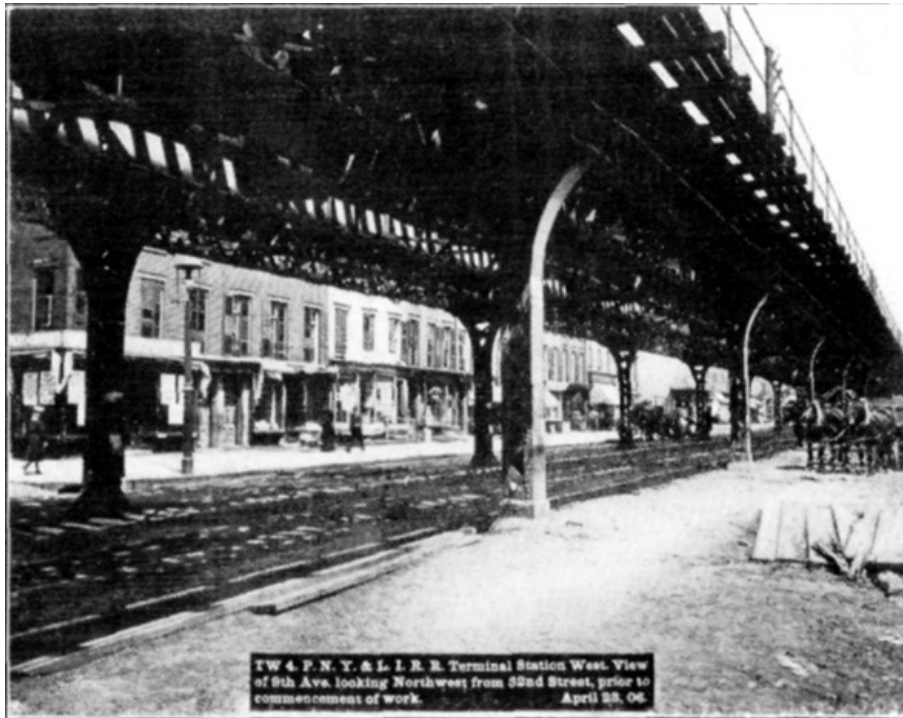
PLATE XLVII, FIG. 1.— TW 4, P.N.Y. & L.I.R.R. TERMINAL STATION WEST. VIEW OF 9TH AVE. LOOKING NORTHWEST FROM 32ND STREET, PRIOR TO COMMENCEMENT OF WORK. APRIL 23, 06.
