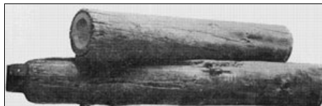
OLD WOODEN WATER MAINS
