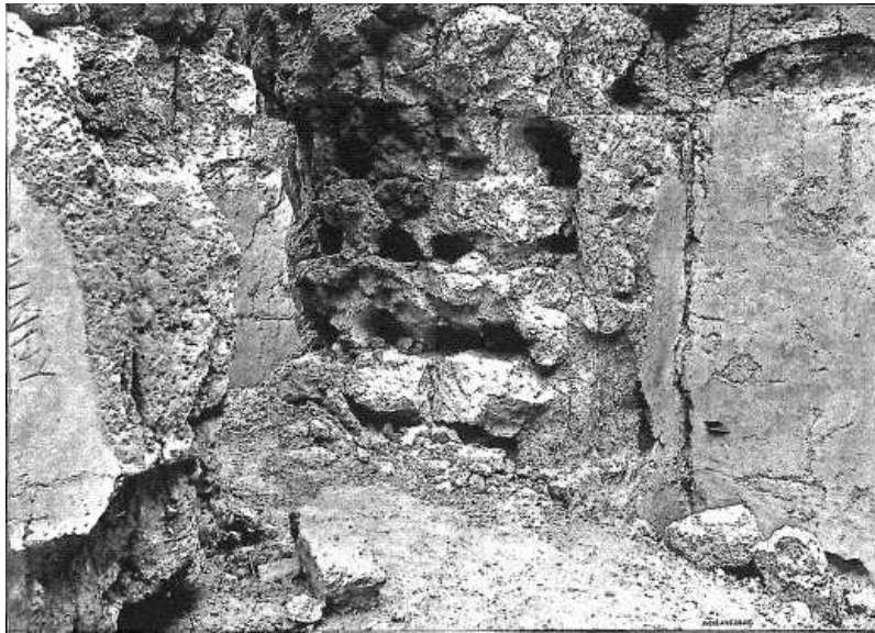
REMAINS OF LINTELS
