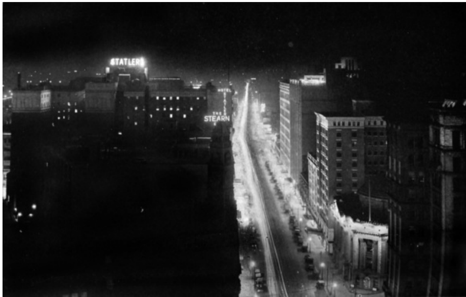
MODERN STREET LIGHTING
