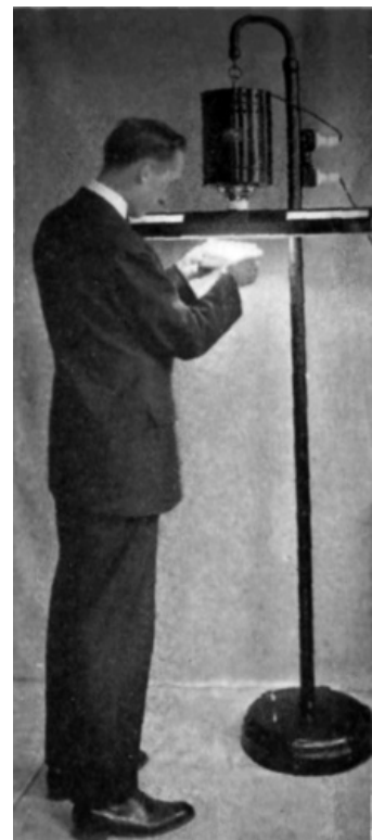
CARBON-DIOXIDE TUBE FOR ACCURATE COLOR-MATCHING
