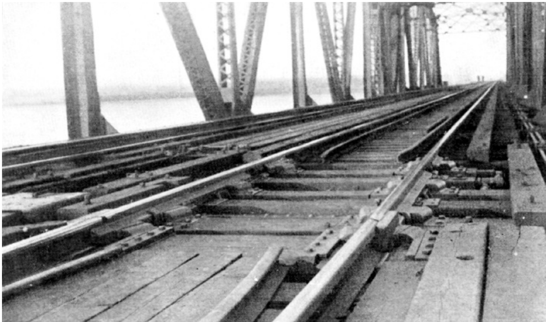
PLATE XX, Fig. 2.—Lift Rail and Locking Device, Draw Closed.
