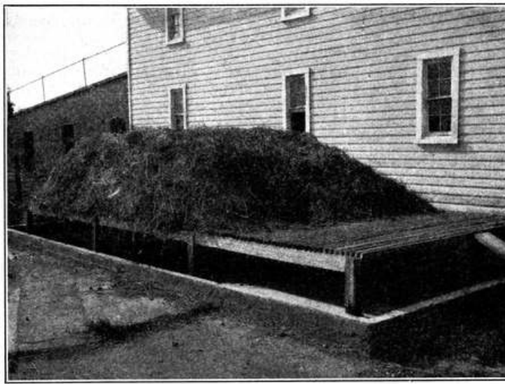
FIG. 9. A maggot trap for house-fly control. View showing the concrete basin containing water in which larvæ are drowned, and the wooden platform on which manure is heaped. (Hutchison.)
