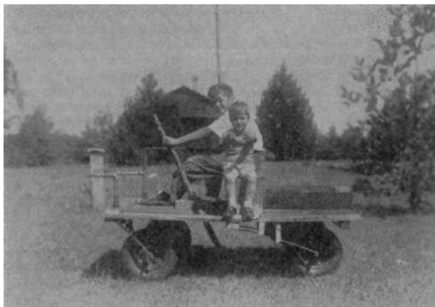
Electrically operated wagon constructed of native butternut wood known for strength and light weight as well as durability. Author's sons aboard. Photo by C. Weschcke 1941.
