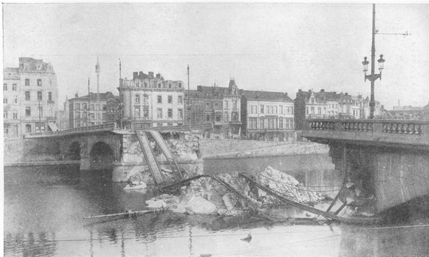
This bridge over the Meuse at Liege was blown up by the Belgians to delay the German advance. The German army crossed on pontoon bridges
