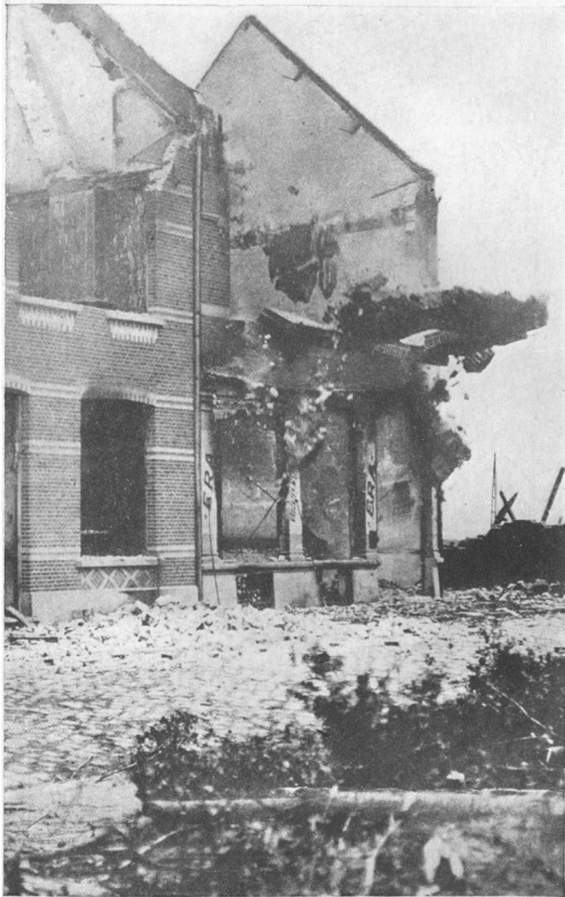
A remarkable photograph taken during the bombardment of Antwerp, showing the falling wall of a house that has been struck by a German shell
