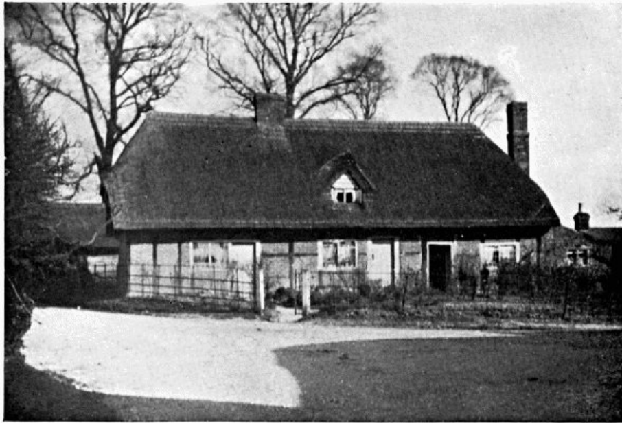
OLD COTTAGES NEAR MACKERY END
