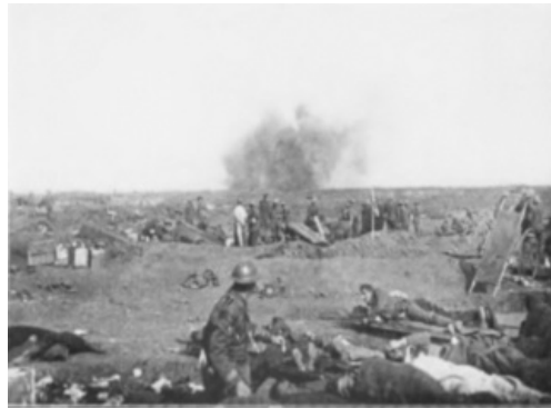
A First Line Hospital
