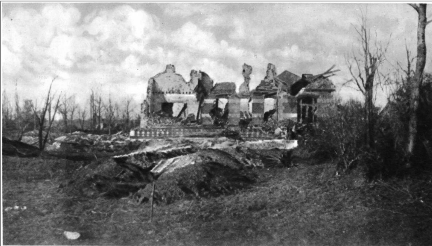
SHELLED, BURNED OUT, AND FINALLY TAKEN BY STORM: ALL THAT REMAINS OF THE FAMOUS CHÂTEAU OF VERMELLES.
