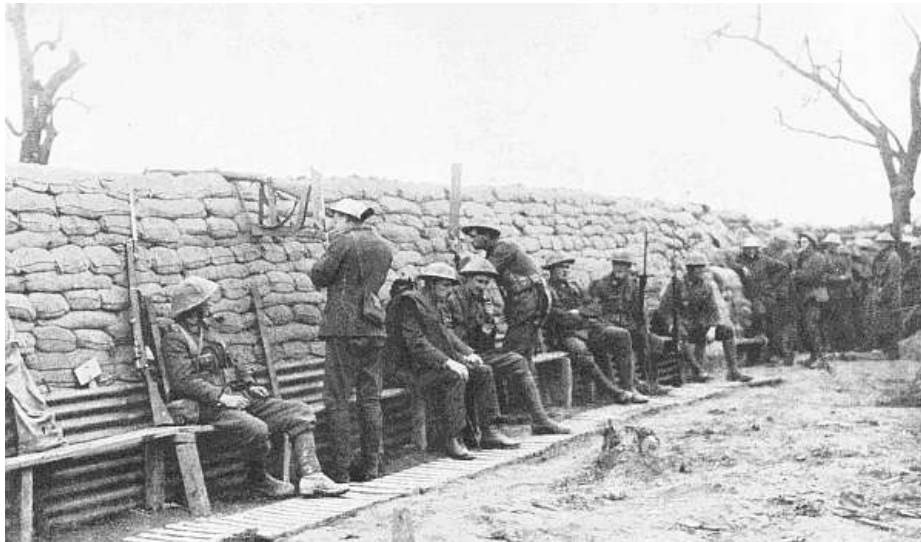
THE TRENCHES HERE HAVE TO BE BUILT ABOVE THE GROUND IN BREASTWORK AND NOT DUG BELOW IT
