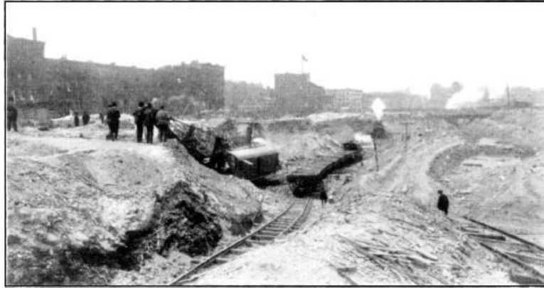
FIG. 2.—EAST PIT, STEAM SHOVEL LOADING EXCAVATED MATERIAL ON CAR.
