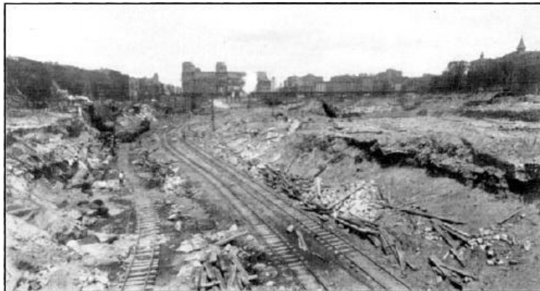
FIG. 3.—WEST PIT, SHOWING CONDITION ON JUNE 28TH, 1905.
