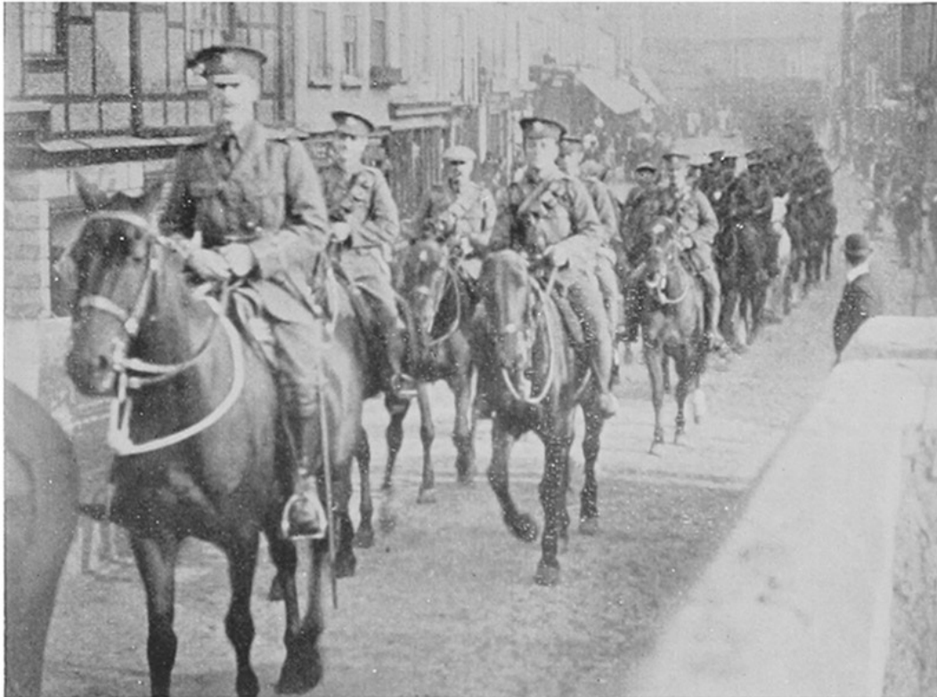
CROSSING THE BRIDGE, ST IVES.
